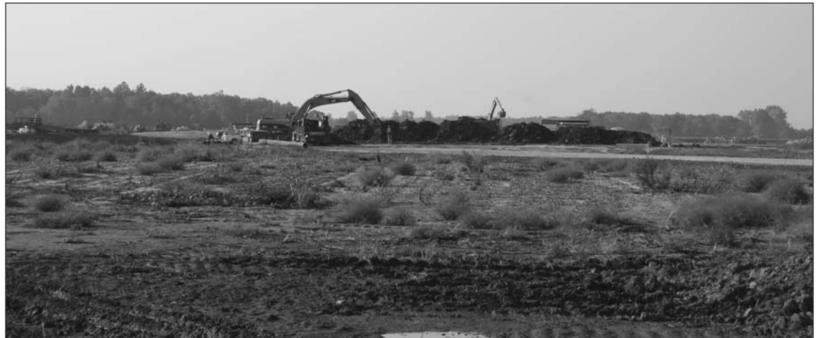
Land north of Urbana is prepared for the new ethanol plant.
