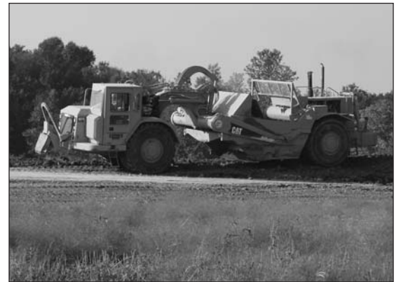
This earth mover prepares ground for construction of the new plant.
